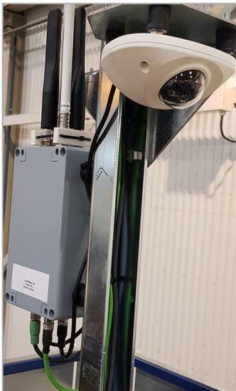
Model-A Router mounted on mast
